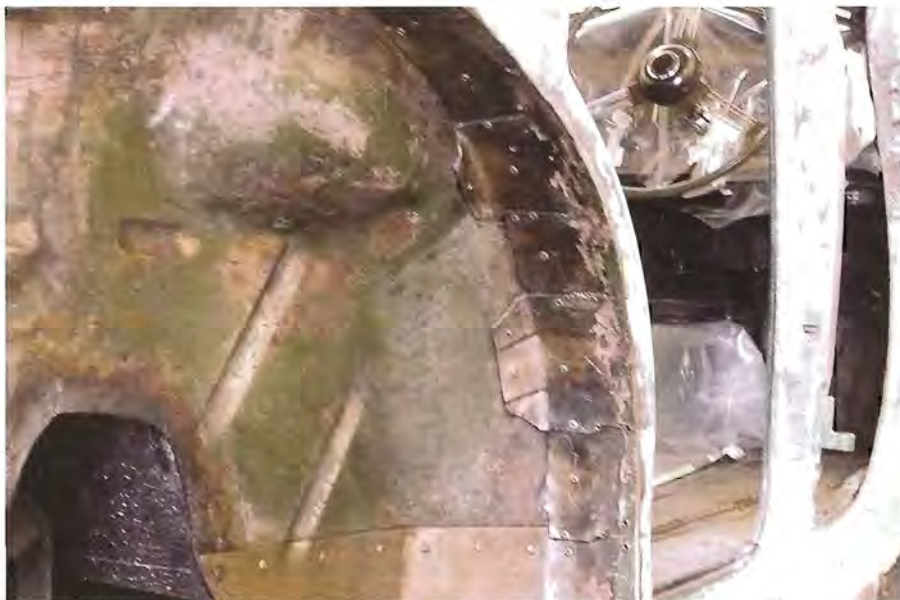
Previous dodgy C Post repairs unearthed.
