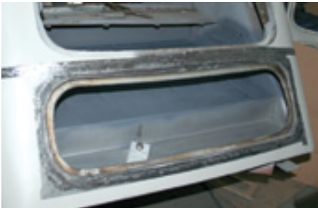
New aperture surround welded into place.
