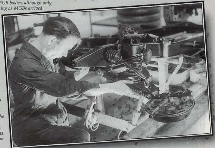
Rear axles are fitted with wheels before they are rolled over to the production line and attached to the chassis. The axle seen here is the type fitted to YAs. Later the YB was to have a more modern, and quieter, hypoid axle.
