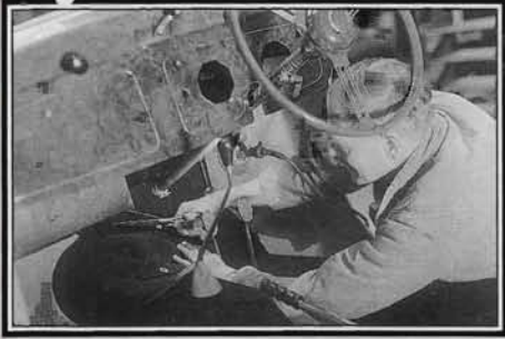
With the bodies in place, the carpet fitter completes his task. Quite a few of the jobs undertaken on the 1947 assembly line needed hand adjustments to make parts fit, unlike modern assembly plants where everything should just slot into place.
