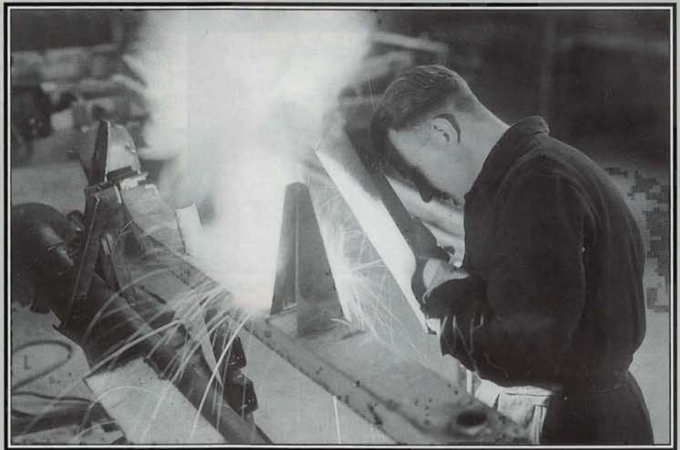
Although Abingdon was always more of an assembly plant than a manufacturer, the chassis frames were built in the press shop right up to the end of MGA production. Here the body mounting brackets are welded on to a Y-type chassis. After completion, the chassis would be painted with 'chassis black' paint and stored until needed.
