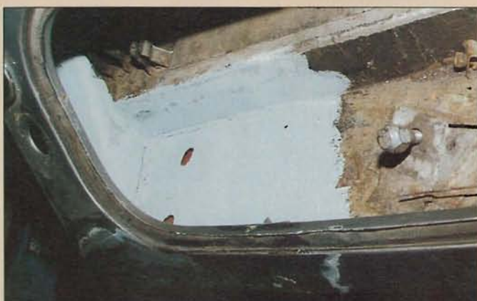
The section of floor replaced in the spare wheel compartment. The body is bolted to the chassis at this point. Note the part-completed work on the panel below the aperture.
